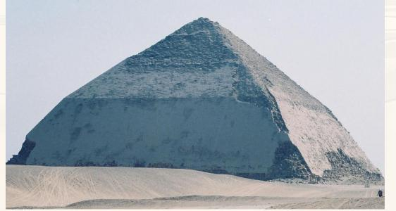
However, when the building began, the 55° angle of the slope was too steep and while building, engineers realised it was unstable. So, half way up, the angle was changed to 43° to make it more shallow.
